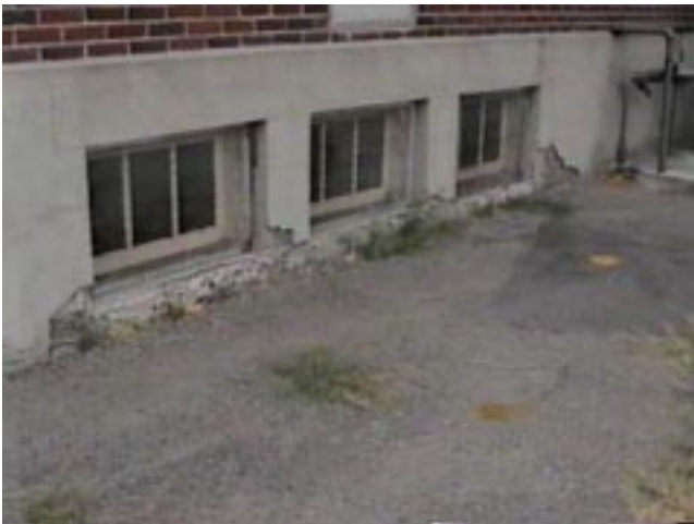
PHOTOGRAPH NO. 7 East side of Garfield Elementary School.
