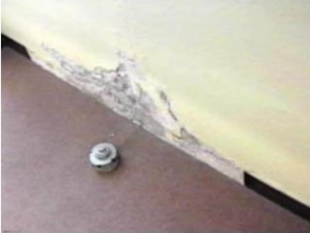
PHOTOGRAPH NO. 6 Clean-out where sewer exits basement of Garfield Elementary.
